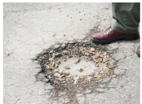
Typical small pothole
